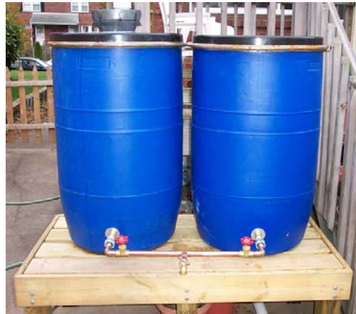
Figure 4: Completed Rainbarrel System
